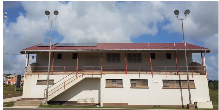
5.0kWp PV System
