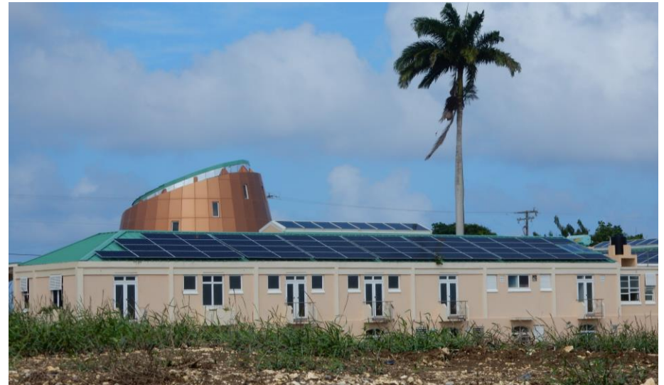
51kWp PV System
